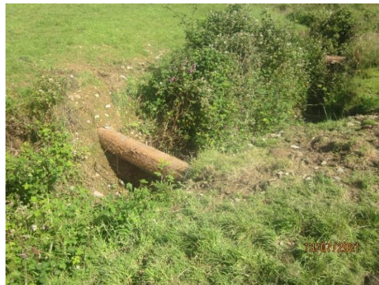
Leaky fence and woody debris dams
